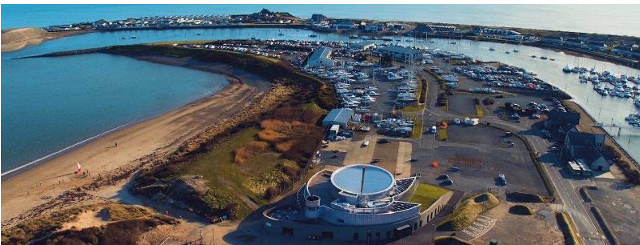
CHPSC at Plas Heli The Welsh National Sailing Academy and Event Centre
